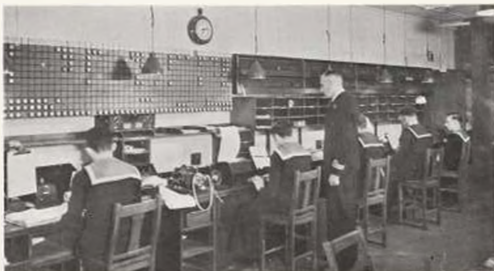
R.T.T. terminal positions for fixed services showing transmitter equipment indicator board
